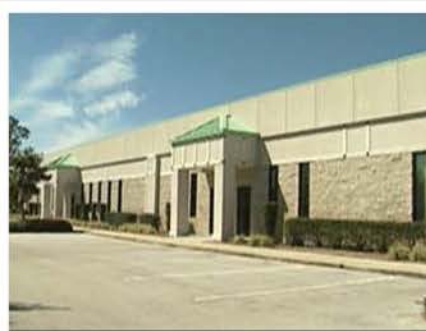
FineTest Building at 1 Industry Drive
