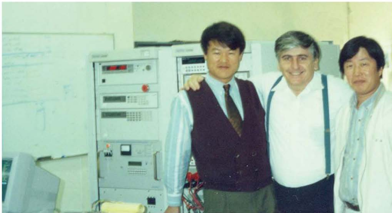
Front view of Tester during Acceptance Test and Training
