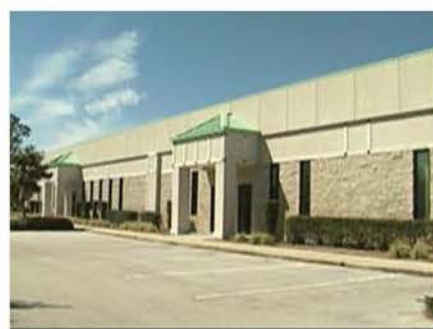
FineTest Building at 1 Industry Drive
